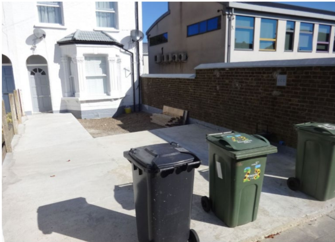
Concrete vandalism in Gypsy Road
